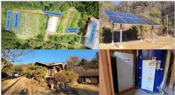
PV + Home ESS (5kW Inverter + BAT)
