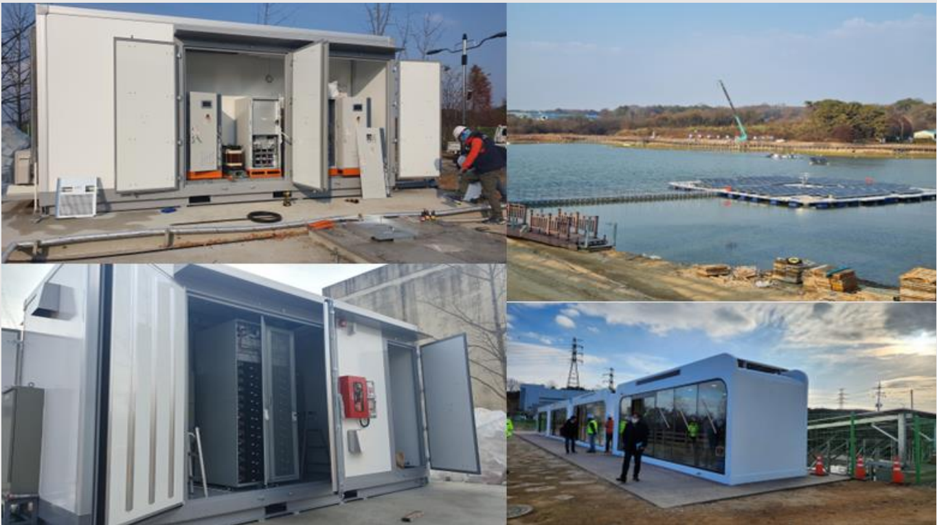
PV + BAT Off-grid DC-ESS (신척저수지)
