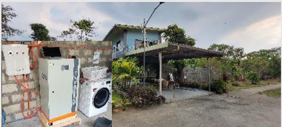
PV + Home ESS (5kW Inverter + BAT)
